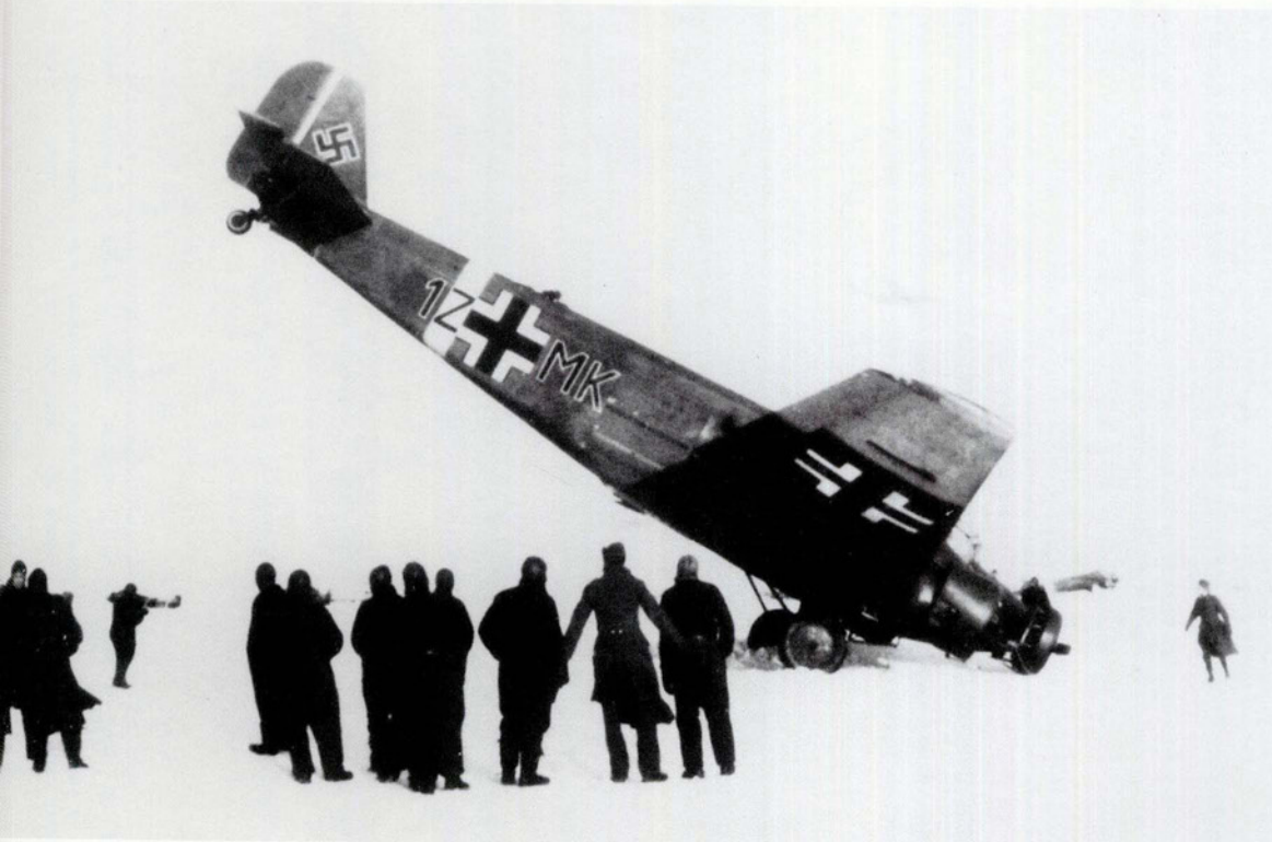
LEFT: With the onset of winter, braking and manoeuvring in the ice and snow was difficult and a good landing was considered quite a feat. This Ju 52/3m, 1Z+MK of 2./KGzBV 1, ended up on its nose after a landing accident at Zaporozhye in late 1941 when the pilot braked too hard. Interestingly, although the numeral 1 appears on the yellow undersurface of the wing tip, indicating that the complete code was painted under the wings, there is no sign of the letter Z, despite the fact that the reflected light from the snow has illuminated the white of the underwing Balkenkreuz. This would suggest that the undersurfaces have been painted later, almost certainly in black. The yellow fuselage band on this aircraft has been applied further forward than was usual.
